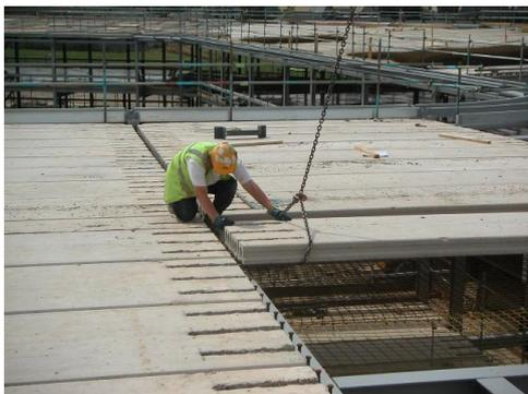
Fig. 1. Precast concrete hollow core slab placed onto steel beams.
