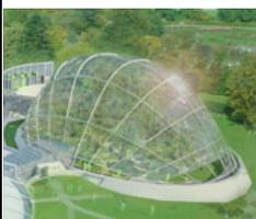
A further example of research directly impacting on industry through a particular building is the 2012 Aarhus Botanical Garden Hothouse in Denmark. Research software based on subdivision surfaces developed by Shepherd was used (with architects C. F. Moller) to design and optimise the design-competition winning building completed in summer 2013, which was shortlisted for two IStructE Structural Awards [6].
