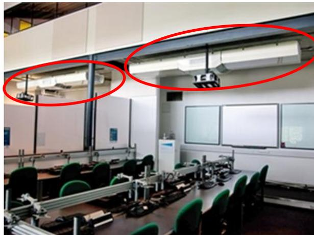
*Figure 2: Two Cool-Phase units mounted on the ceiling of an ICT suite in the University of East London*
